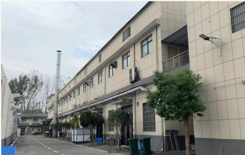
Main Production Workshop Building
